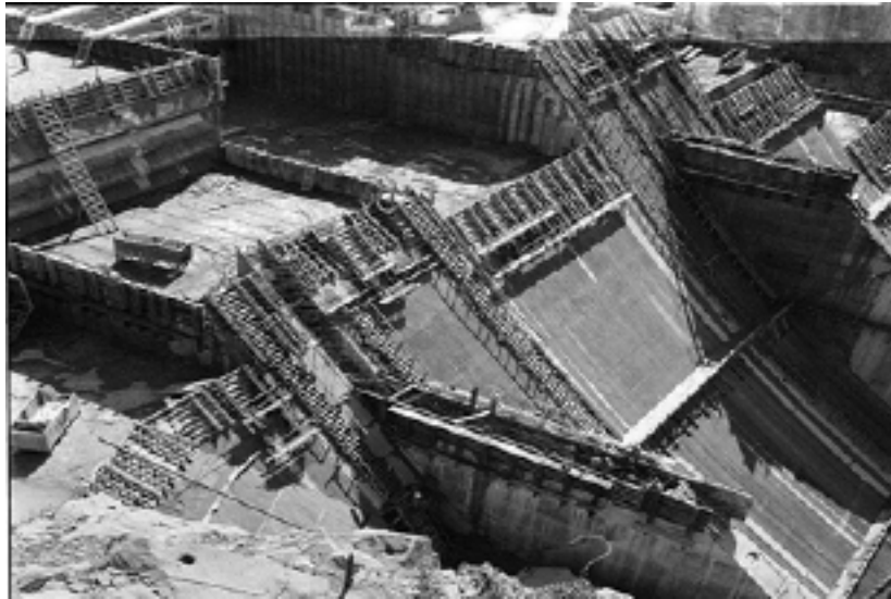
Fig. 3.2.4 The Bhakra-Nangal Project under construction in 1960
