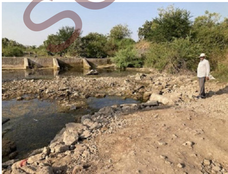
Fig. 1.1.6 A community-managed check dam built on a stream passing through Pransla village in Gujarat
